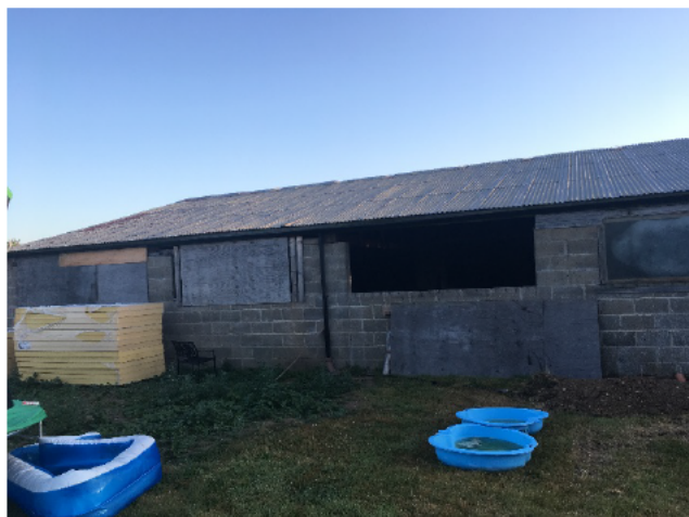
Photo 7. Poplar Farm – southern elevation of Mr Durrant's barn showing open window opening and breeze block construction with sheet metal roof.
